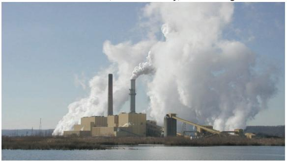
Kentucky Utilities coal-fired Ghent power plant in Carroll County had a net generating capacity of 2,000 megawatts in 2006. Each of Ghent's four generating units can produce enough electricity to light 5 million 100-watt light bulbs. The station consumes an average of 14,000 tons of coal daily. Gypsum from plant scrubbers is processed and shipped to nearby BPB plant and used for manufacturing wallboard. Photos by Dan Carey, Kentucky Geological Survey.
